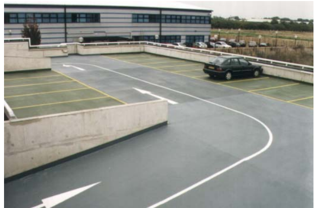
A car park structure subjected to a comprehensive concrete repair and deck waterproofing scheme devised and administered by Sandberg
