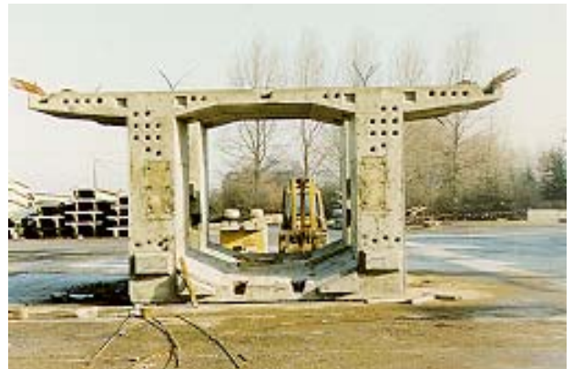
Inspection of post-tensioned glued segmental viaduct unit
