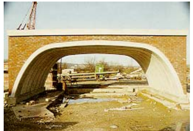
Inspection of precast concrete arch bridge unit
