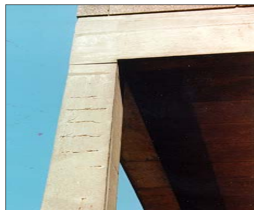
Reinforcement corrosion
