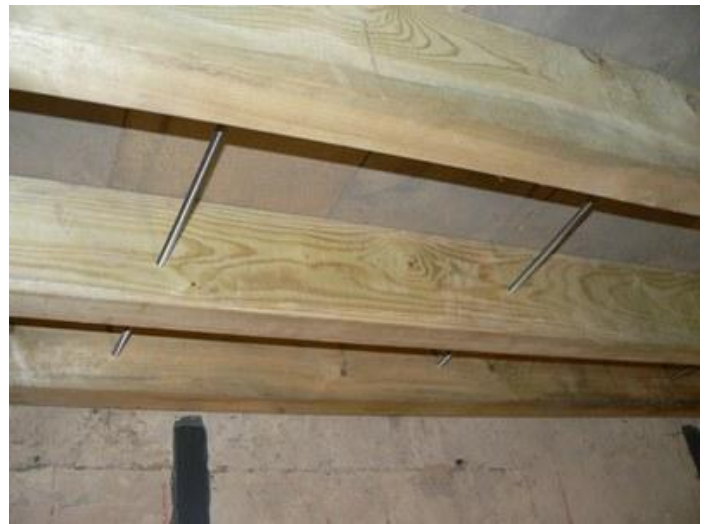
Figure 8. Helical stainless steel fixings to restrain gable wall
