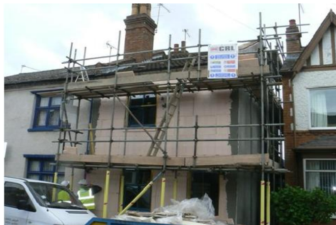
Figure 7. Rendering removed and insulated cladding being installed
