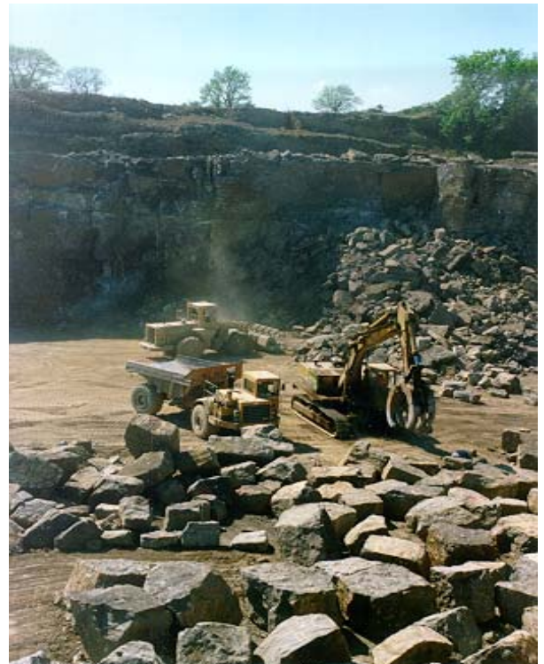
Stockpiling of large armour units in a quarry
