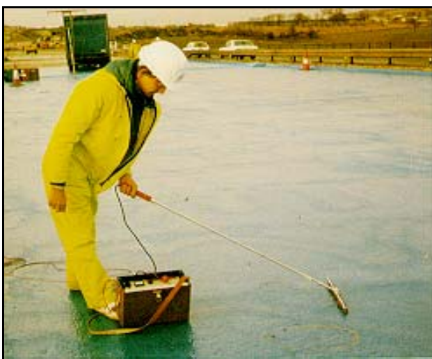
Quality control checking of bridge deck waterproofing using high voltage techniques
