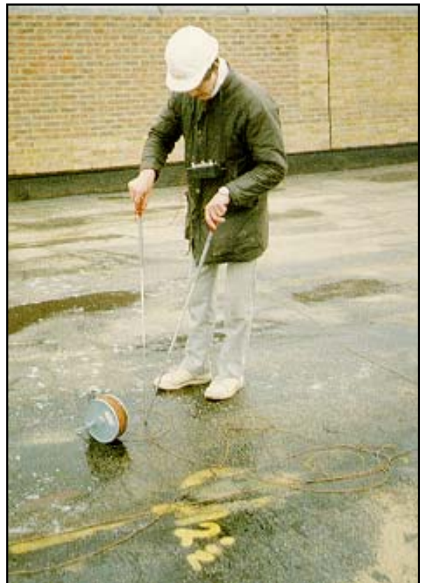
Low voltage equipment being used to check a waterproof membrane
