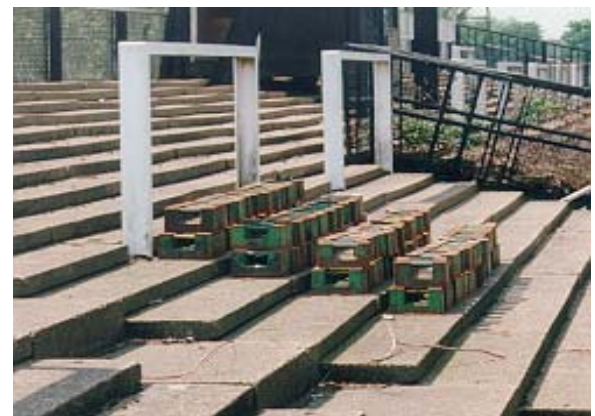
Kentledge on precast concrete planks
