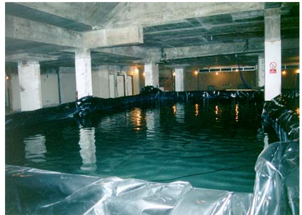
Part of a 150 tonne load test
