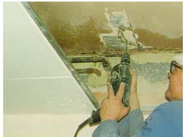
One sampling technique with minimised damage and disturbance
